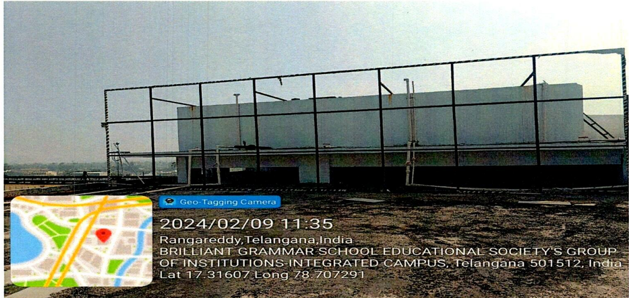
Over head tank at Block - I
